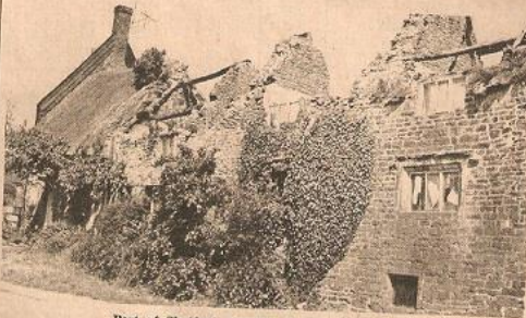
Part of Shutford, showing derelict Cottages.
