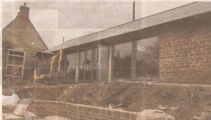
Shutford village hall is just months away from completion
